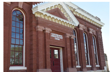
Renovated Galveston Water & Electric Light Building
