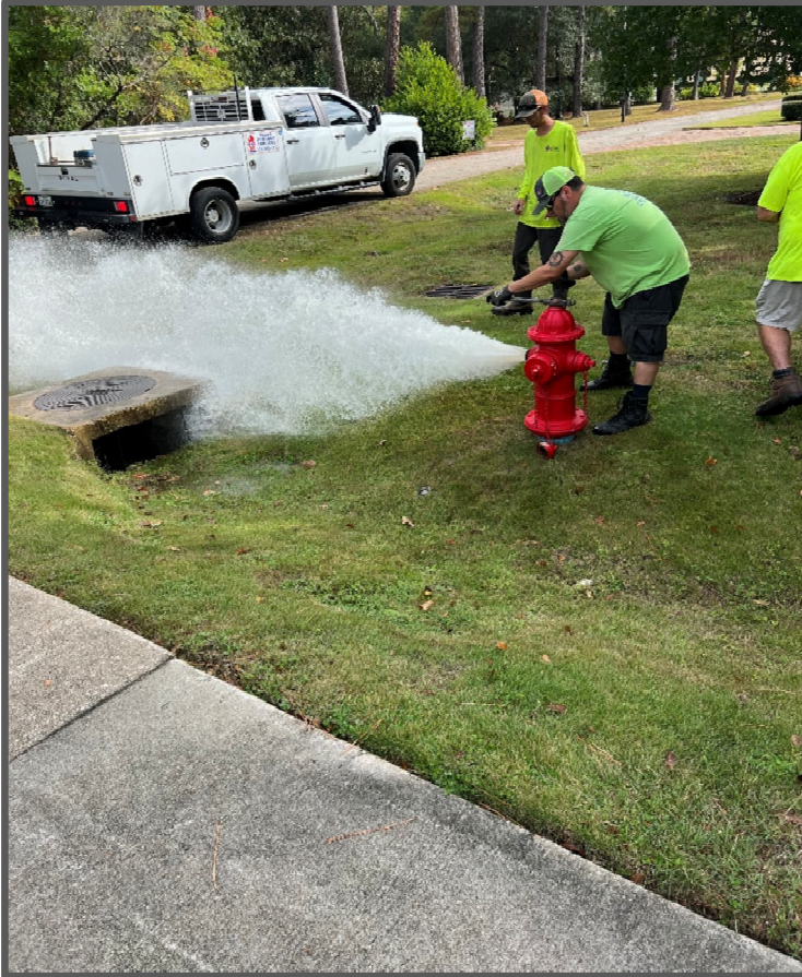
Fire Hydrant Field Testing
