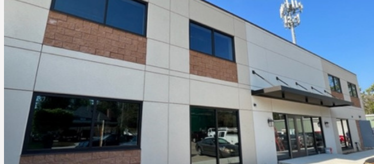
Public Works & Disaster Operations Building
