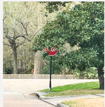
Example of vegetation obstructing a stop sign
